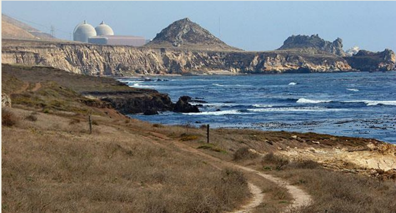
The Diablo Canyon nuclear power plant on the coast outside San Luis Obispo, California Michael A. Mariant/AP
